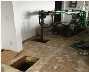
A helical pier machine sets a pier to stabilize the center of the house.
